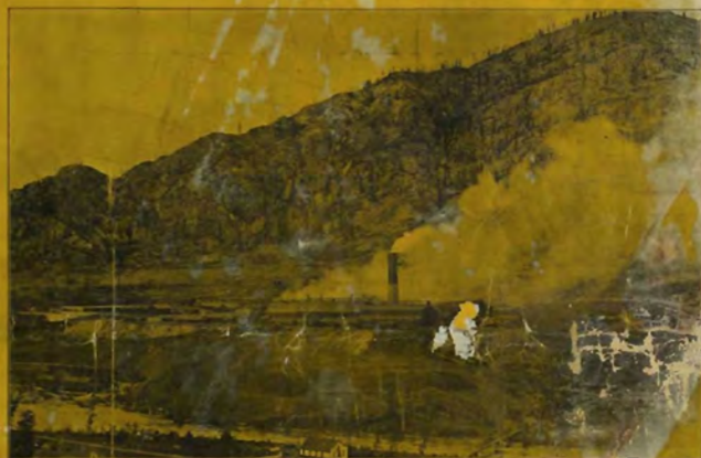
GRANBY CO.'S SMELTING PLANT, KAND. OKS, B.C. Capacity, 2,000 tons daily.
