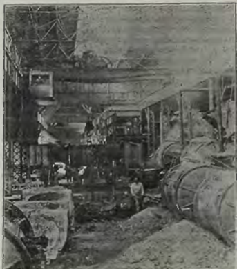
CONVERTER ROOM AT GRANBY SMELTER.
