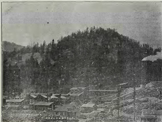
BRITISH COLUMBIA COPPER CO.'S MOTHER LODGE MINE, 1904.
