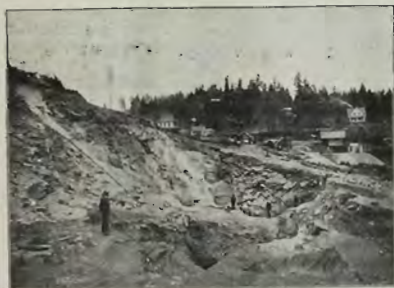
ORE QUARRY, SHOWING MOUTH OF RAISE.
