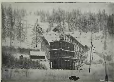
RAWHIDE MINE, SHOWING TRAMWAY AND ORE BINS.
