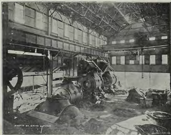
BRITISH COLUMBIA COPPER CO.'S CONVERTER ROOM.
